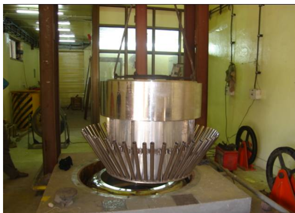
Install and Operate Irradiator being installed.
