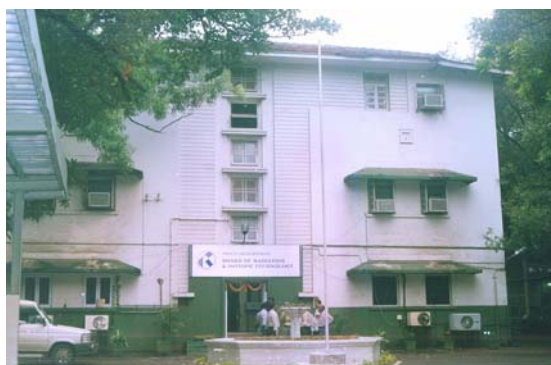
Project House at Anushaktinagar where CSSC is located
