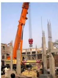
IFRT Hot Cell under Construction
